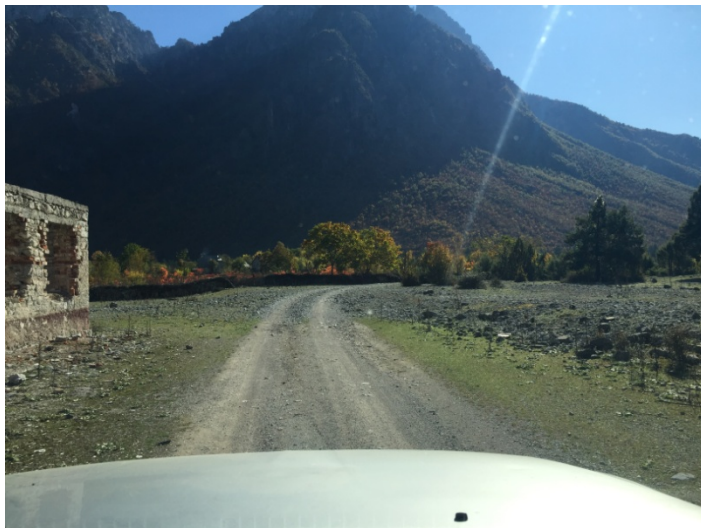
Km 6+960 fundi i rruges
