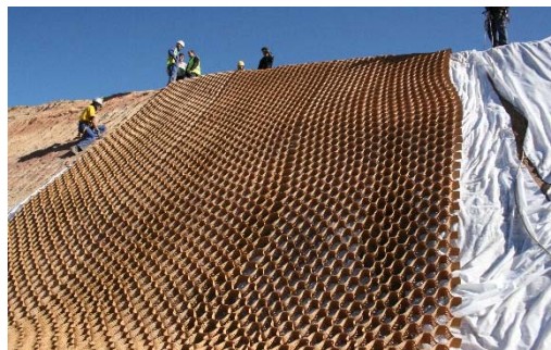
FIGURE 1 - INSTALIMI I GEOCELL
