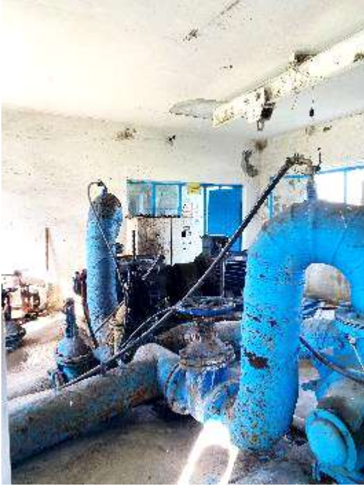
Pompa e cila dergon ujin ne depot e njesive administrative
