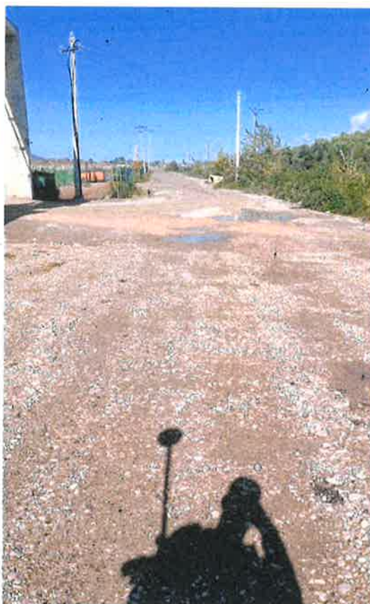
Vazhdim Rruga Uillon
