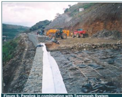
Figure 9- Paralink in combination with Terramesh System
