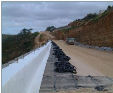
Figure 8 - Paralink in combination with Terramesh System
