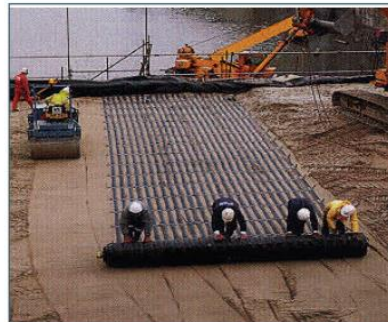
Figure 10- Paralink in combination with Terramesh System
