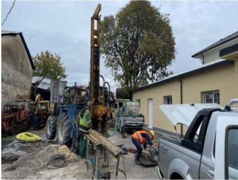
Photo no.5 View from drilling at BH-2
