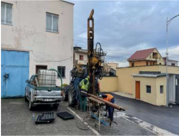
Photo no.1 View from drilling at BH-1
