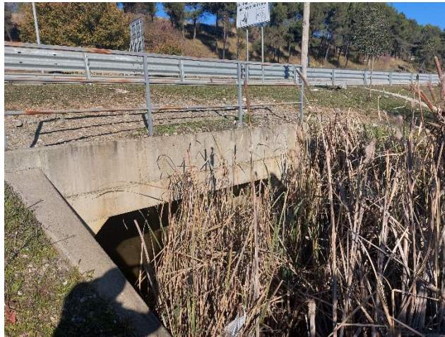
Figura 1-2 C_01, Box Culvert (4m x 2m)
