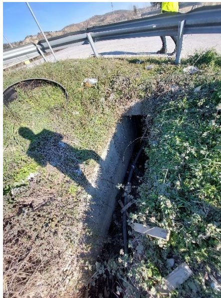
Figura 1-21 C_25, Box Culvert (4m x 1m)
