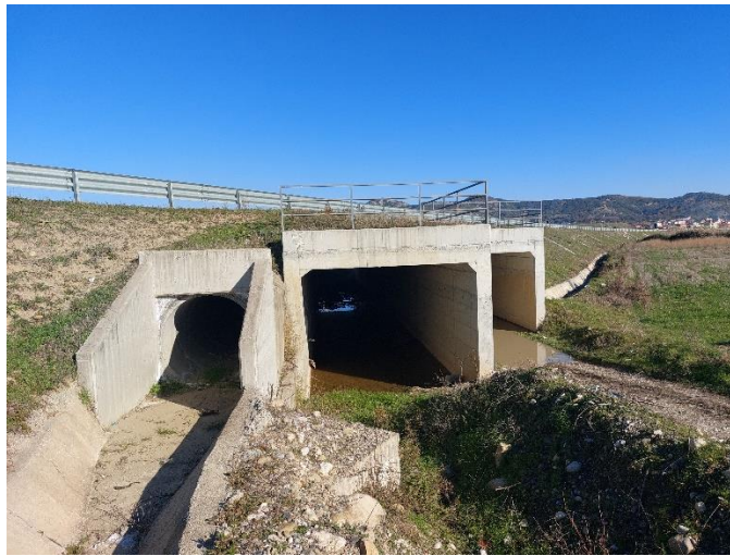
Figura 1-9 C_08, Tombino (D= 1500mm), Double Underpass (4m x 2.5m)
