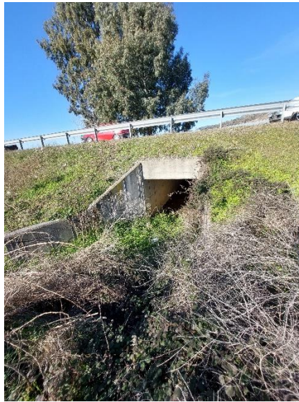
Figura 1-20 C_24, Box Culvert (2m x 2m)
