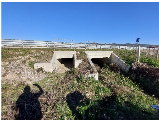
Figura 1-12 C_11, Box Culvert (1.5m x 1m), Box Culvert (4m x 2m)
