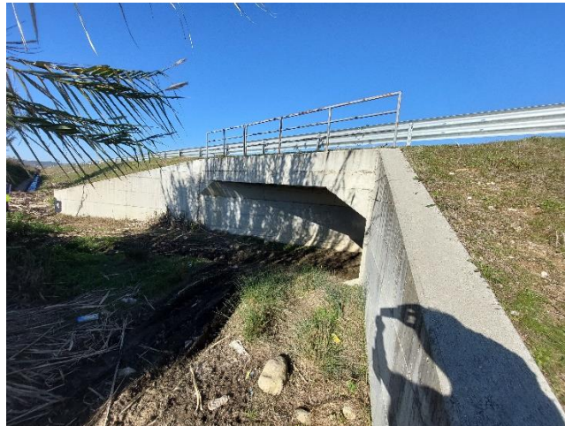
Figura 1-15 C_13, Box Culvert (4m x 2.5m)
