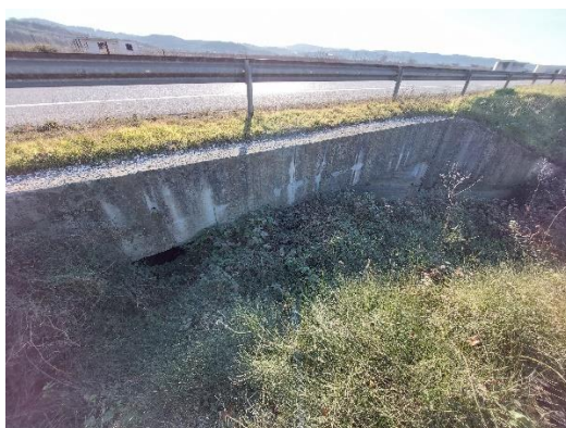
Figura 1-29 C_33, Box Culvert (5m x 2m)
