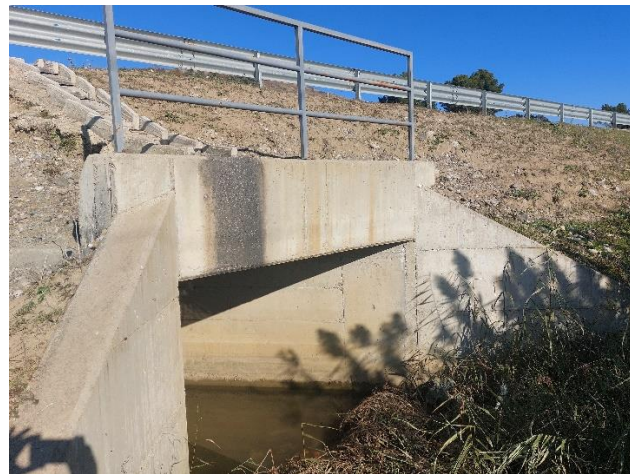
Figura 1-3 C_02, Box Culvert (2m x 2m)
