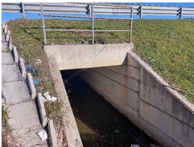
Figura 1-7 C_06, Box Culvert (2m x 2m)
