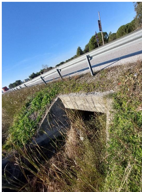
Figura 1-27 C_31, Box Culvert (2m x 2m)
