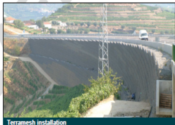
Terramesh installation
