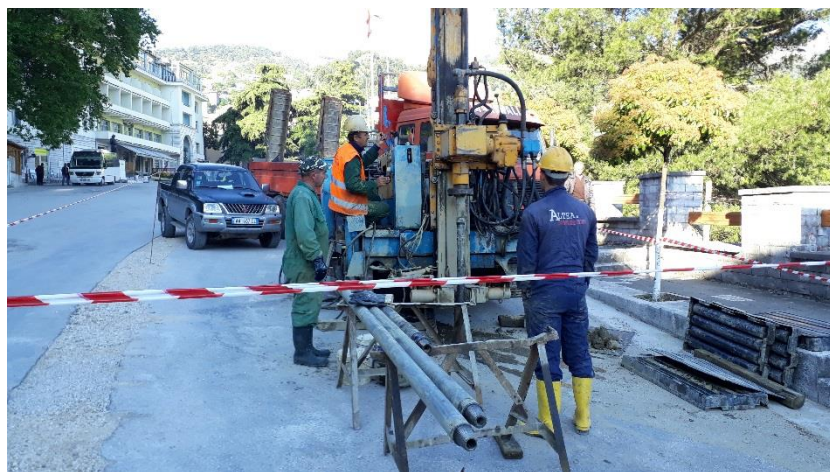
Photo no.1 Location of the drill rig at BH-4
