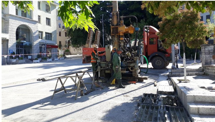
Photo no.1 Location of the drill rig at BH-5
