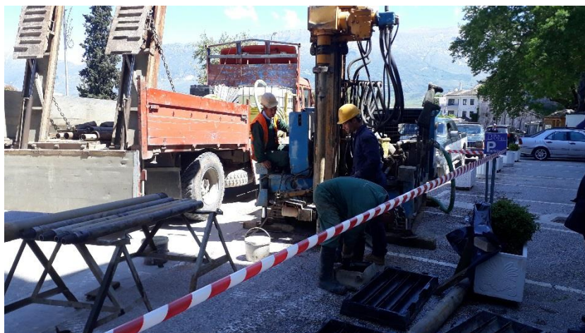
Photo no.1 Location of the drill rig at BH-1
