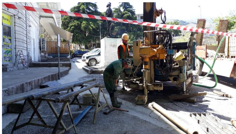
Photo no.1 Location of the drill rig at BH-2
