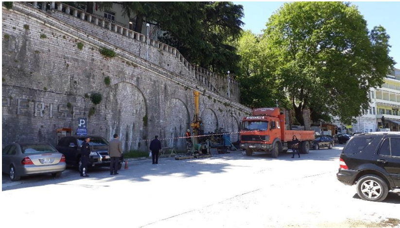
Photo no.1 Location of the drill rig at BH-3
