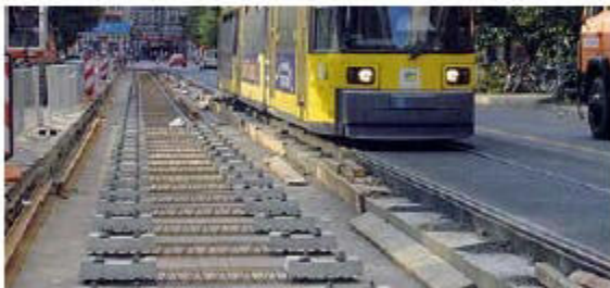
Final installation and fixing of the track panel
