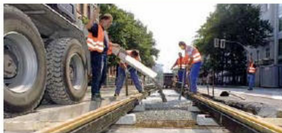
Concreting of the track panel
