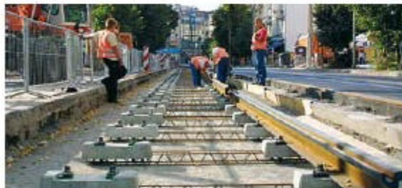
Concreting of the track panel
