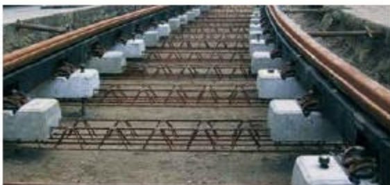
Final installation and fixing of the track panel
