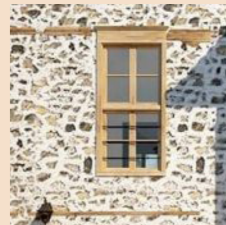
Stone wall with white mortal
