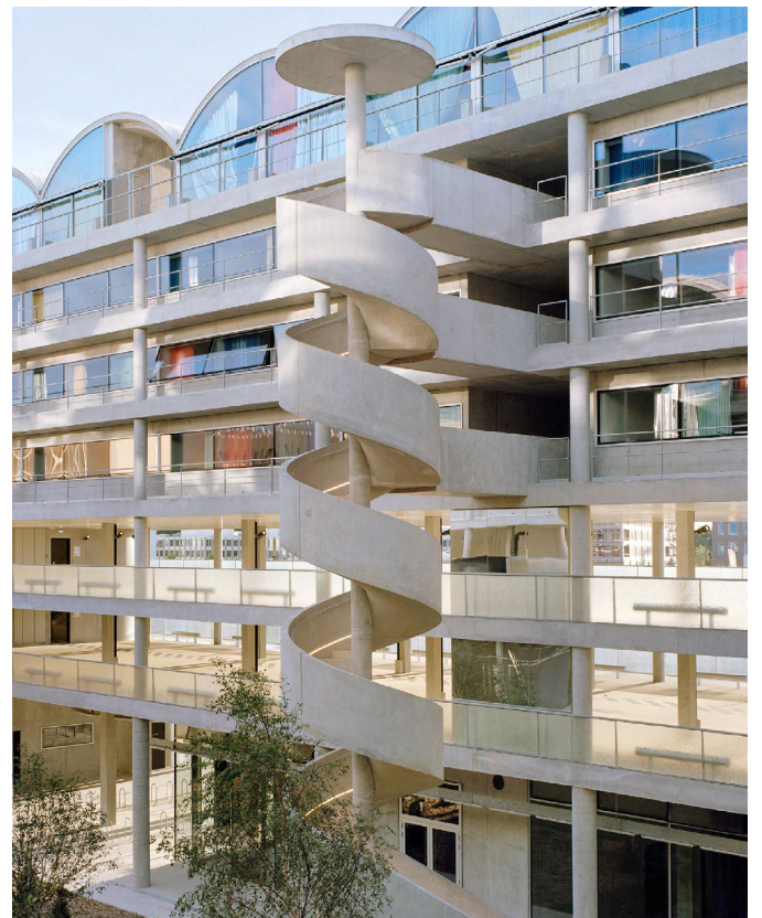
Concrete Stairs for the fire scape in the north
