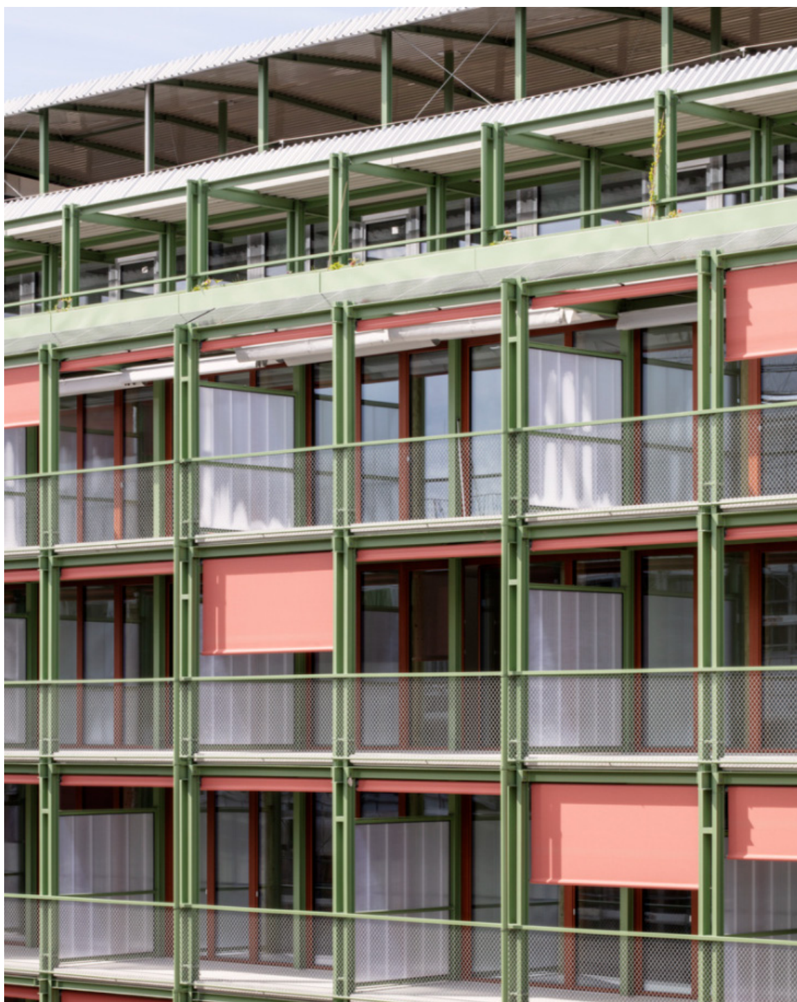
Shades placed in the façade.
