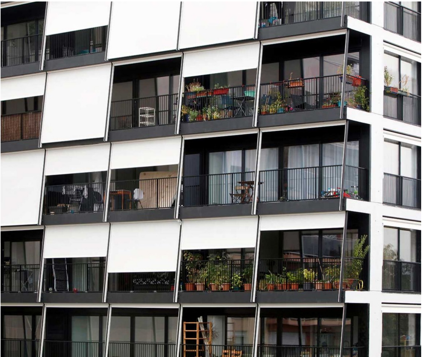
Balconies and shades for the South façade
