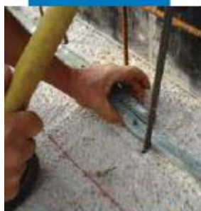
Fixing Idrostop B25 in place
