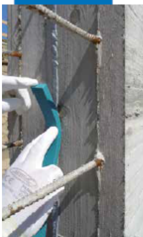
Applying Idrostop Soft on vertical surfaces
