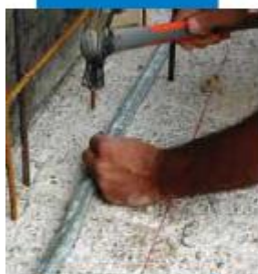
Fixing Idrostop B25 in place
