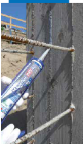
Extruding Mapelflex MS45 prior to applying Idrostop Soft in second pours
