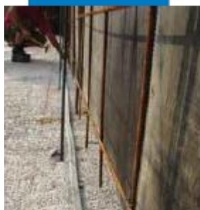
Laying Idrostop B25
