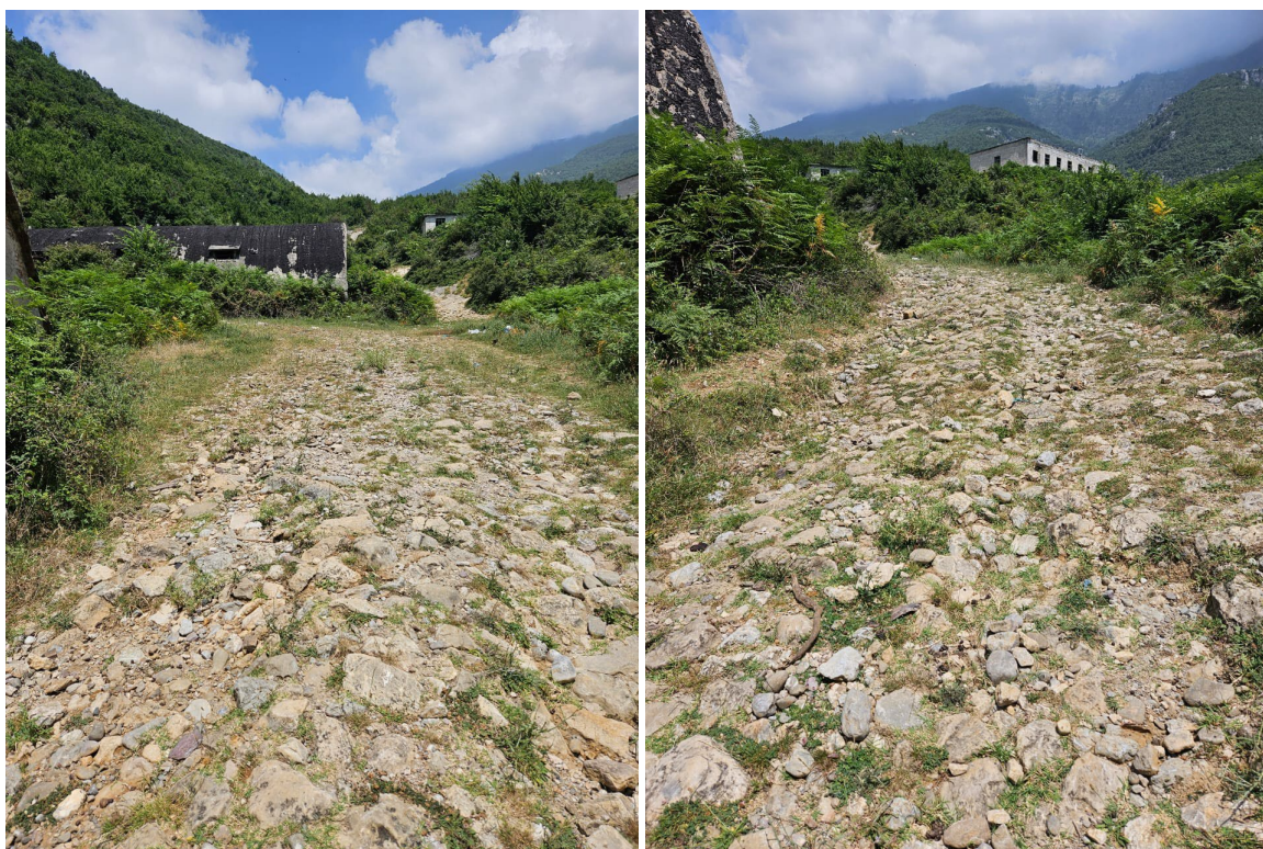
Figure 15 Rruga pergjate progresivit 0+340
