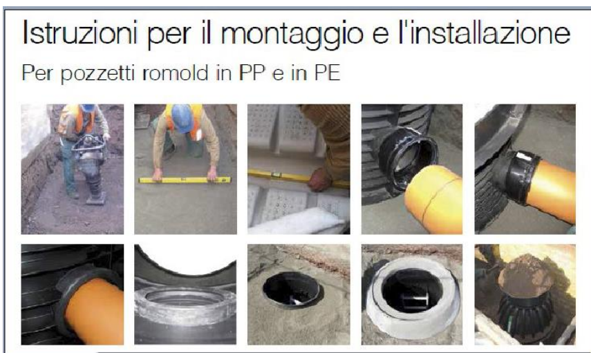
Figure 4.6 Detaje te montimit te pusetave teknike
