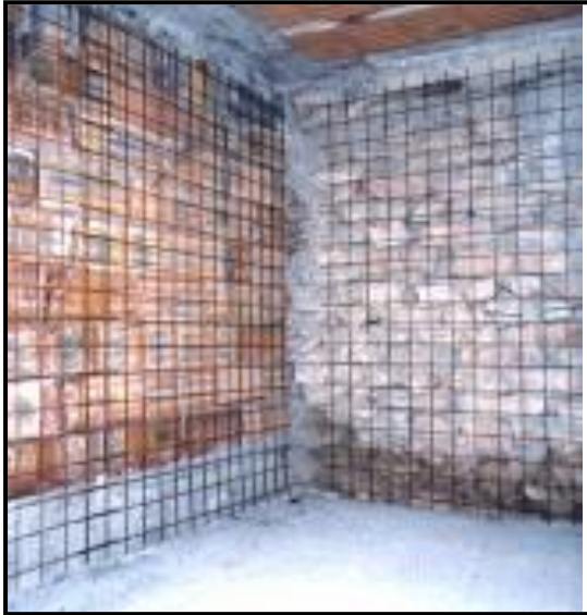
Fig. Ilustrime te perforcimit me kemishim te mureve
